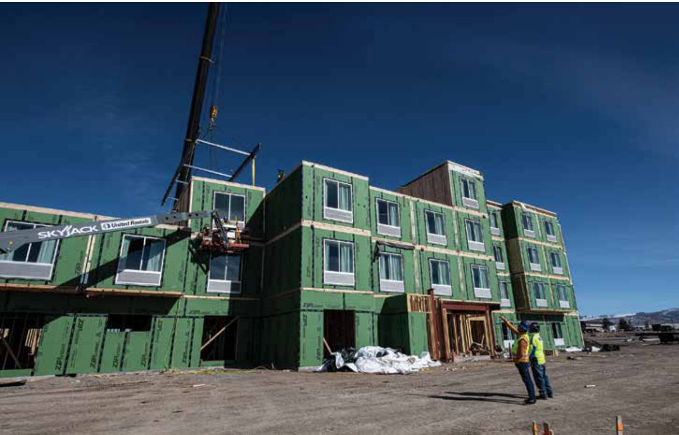
Marriott Hotel modular construction in progress.
